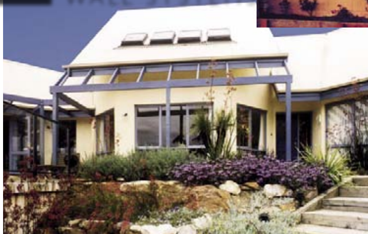
*The Outlook – Award Winning 5 Star Energy Efficient Home using CSR Hebel Block Wall System, Designed by Ecological Architect Gareth Cole – www.garethcole.com
