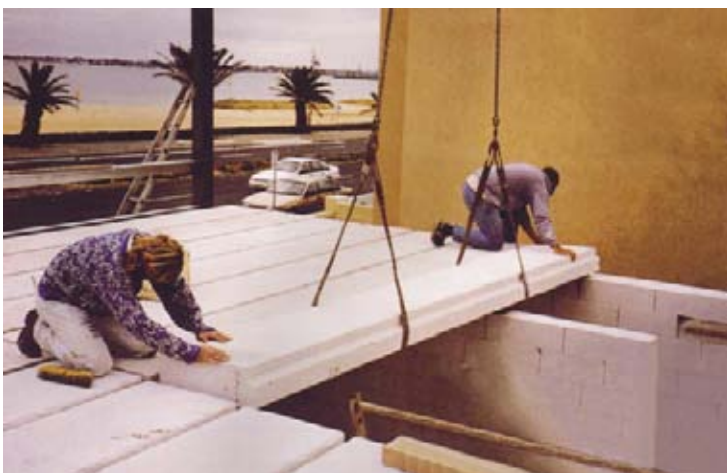
CSR Hebel Panel Floor Systems speed construction time and provide an excellent platform for laying all types of floor coverings.
